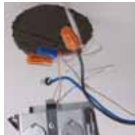
The Halo Slide-N-Side™ wire traps let you make all wiring connections outside the junction box.
