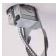
Insert plaster frame into ceiling opening.
