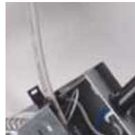
Slide cable into Slide-N-Side™ wire trap and close junction box cover.
