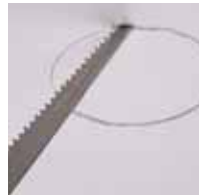
Cut hole in ceiling using template supplied.
