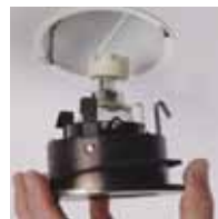
Insert trim to complete installation.
