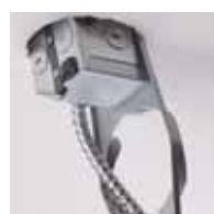
Insert plaster frame into ceiling opening.
