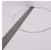
Cut hole in ceiling using template supplied.
